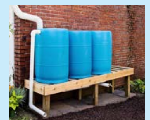
Rain barrels capture water and reduce runoff, lowering the demand for municipal water supplies. Copyright © 2020 Edmonton Food Council
