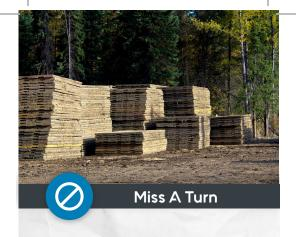
Soil tests show sensitive areas. Need to order rig mats so equipment does not damage the soil.
